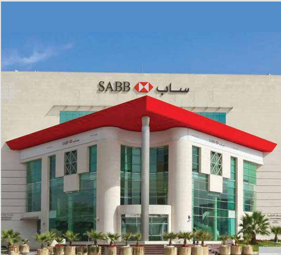
BRANCH SIGNAGE & RED CANOPY CLADDING
